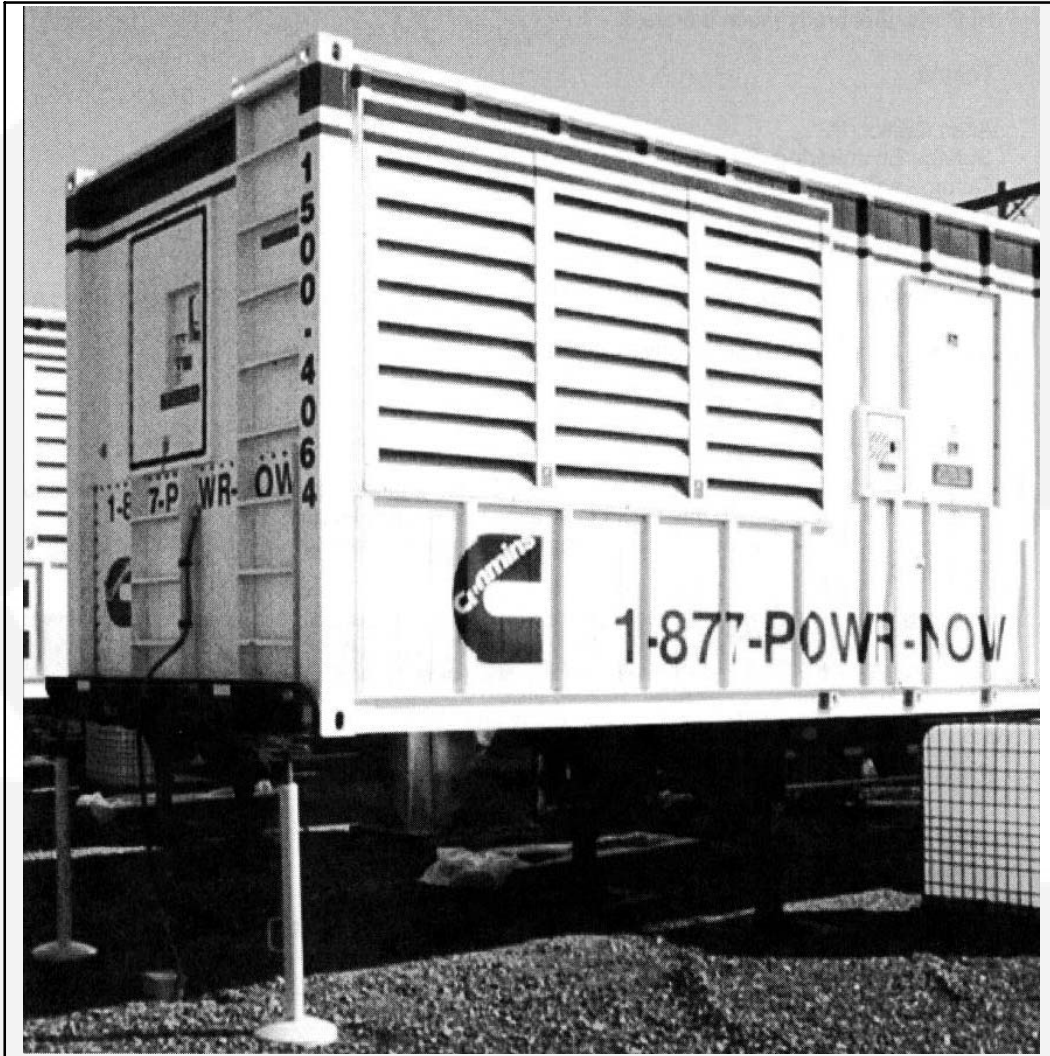
Jack Stands at Nose of Container
