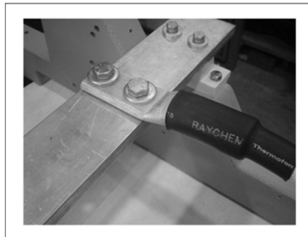
FIGURE 19. CORRECT CABLE CLAMPING (SINGLE LOAD CABLE)
