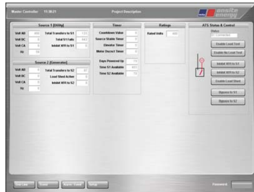
Automatic Transfer Switch
