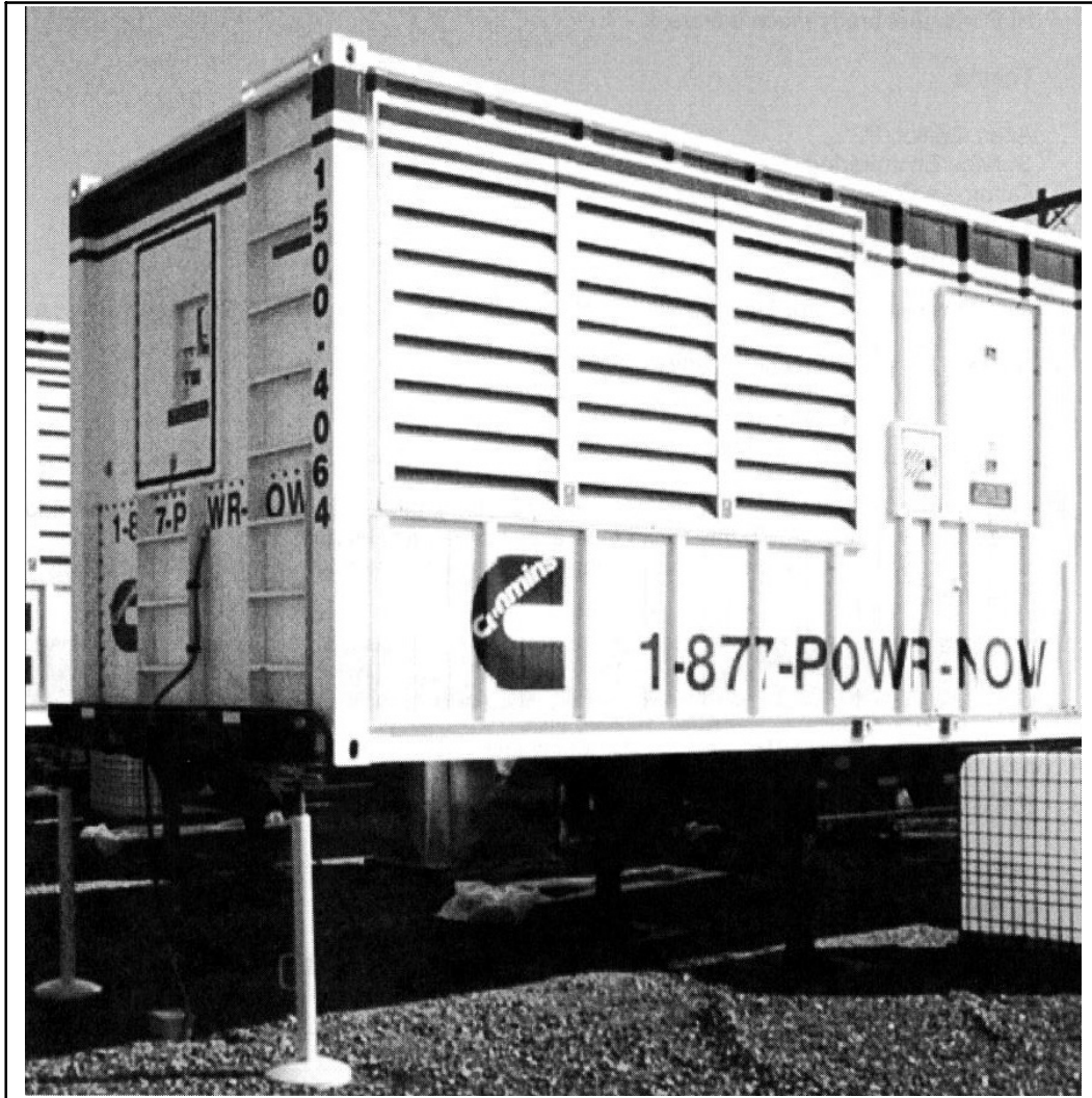
Jack Stands at Nose of Container
